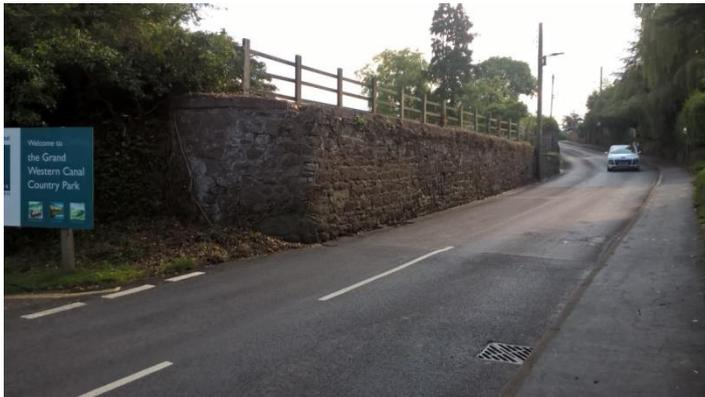
It is expected to take nine weeks to remove the existing wall, dig out the tons of earth behind it, build a new retaining wall, and to create the new pavement. A temporary telegraph pole has been installed to preserve the power supply to the Duck's Ditty floating café-bar whilst the underground cables are disconnected. The new concrete wall will be faced with stone from the existing wall so that the historic
