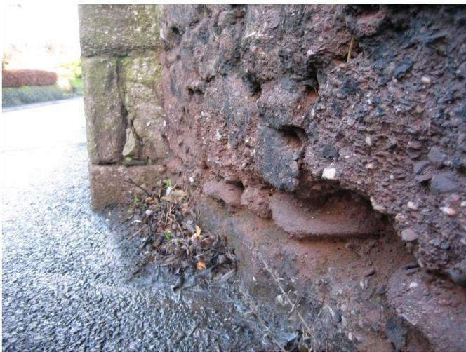
There is also a gradually worsening problem with the wall between the garden of The Moorings and the road. Spray from cars is slowly eroding the soft breccia stone and undermining the wall along the bottom 40cm. Corporate funding has been secured to address this issue by installing a kerb and adding a shoulder of cement to protect the bottom courses of the wall from further erosion. This work will be undertaken whilst the current road closure is in effect in order to avoid further disruption.
